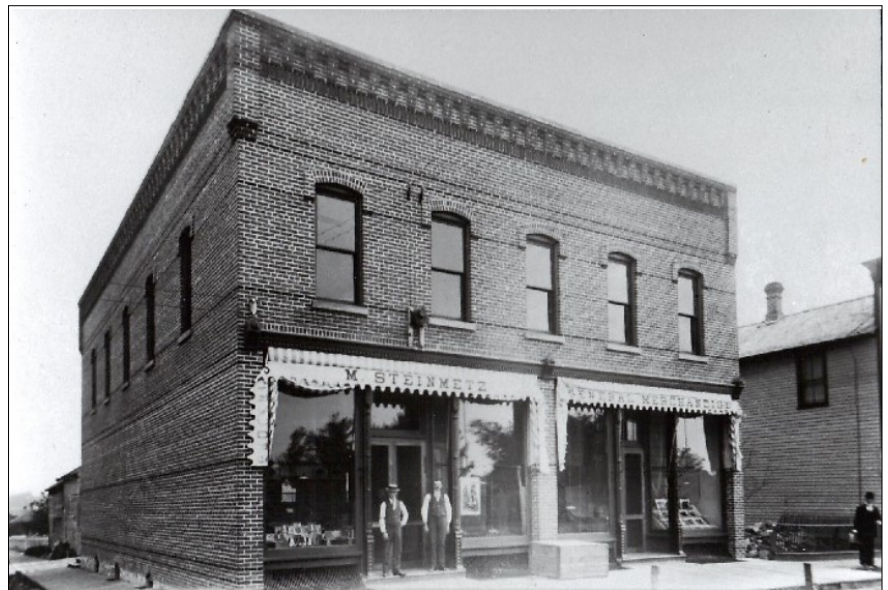
M. Steinmetz General Store located on the southeast corner of A Street and Central Avenue, 133-135 North Central Avenue, ca. 1892. (photo from the North Wood County Historical Society)
